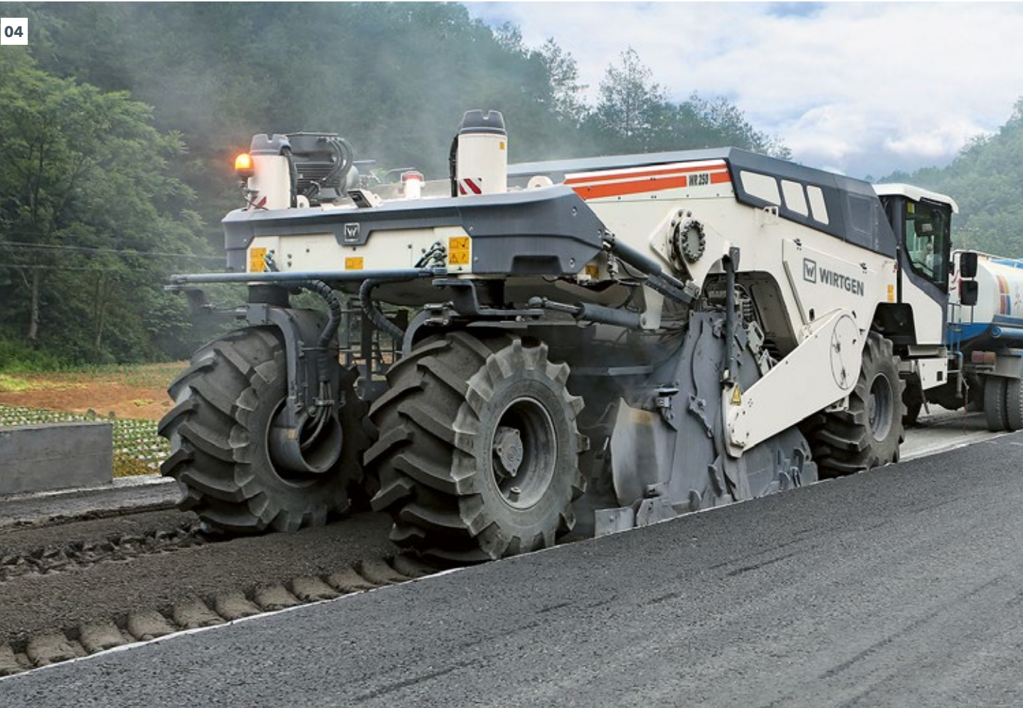
01 - 04 In cold recycling, damaged asphalt layer are granulated, mixed with binding agents, processed, compacted, and repaved.
